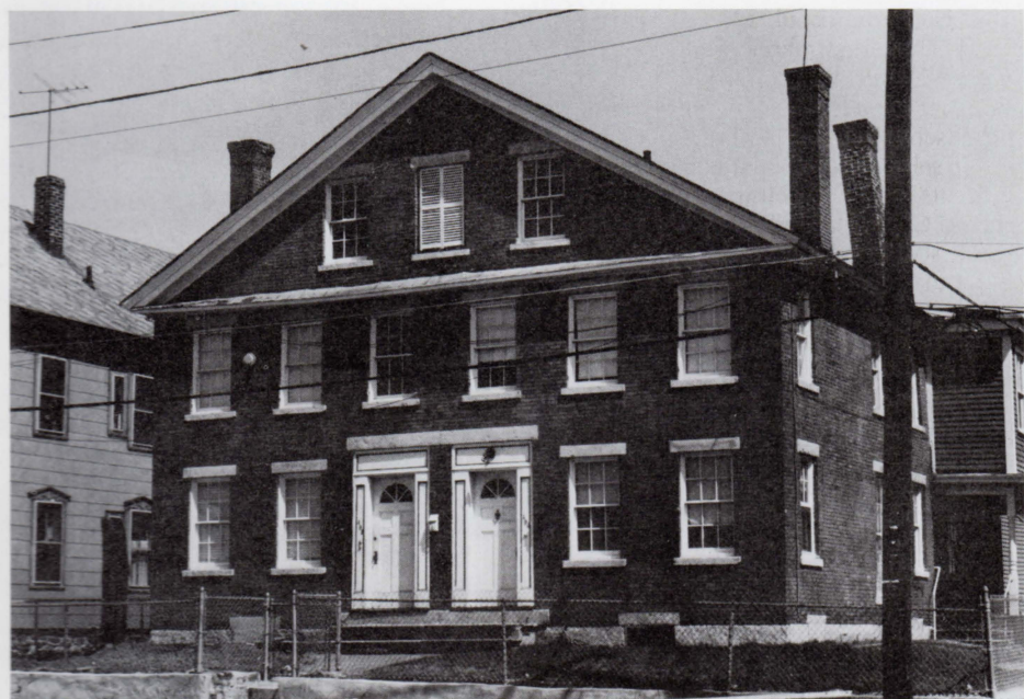
13. 492 Gorham St., 1840s. Broad-gable double houses made of brick are not as common as those of frame construction. Located at the terminus of the Lowell Connector, this handsome Greek Revival residence has retained its double entrance with side pilasters and shared granite lintel, tall end chimneys, boldly articulated pediment, granite trim and six over six sash.
